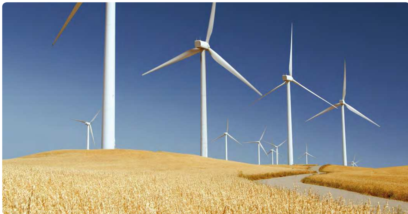
Wind turbine generator
